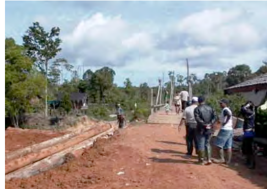
Bridge Construction on the road leading to the Land
